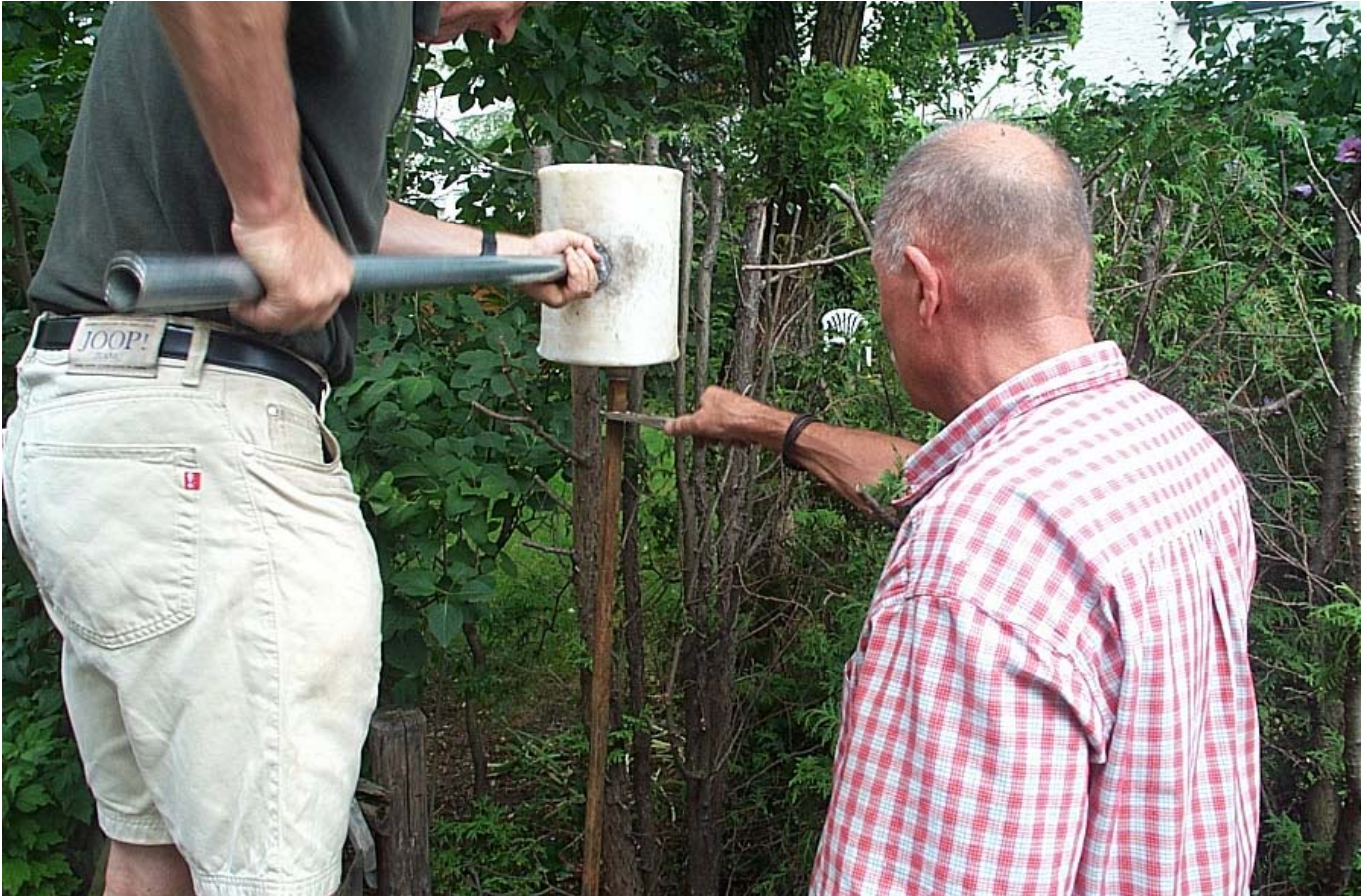
Driving of small-diameter installation casing into borehole.
