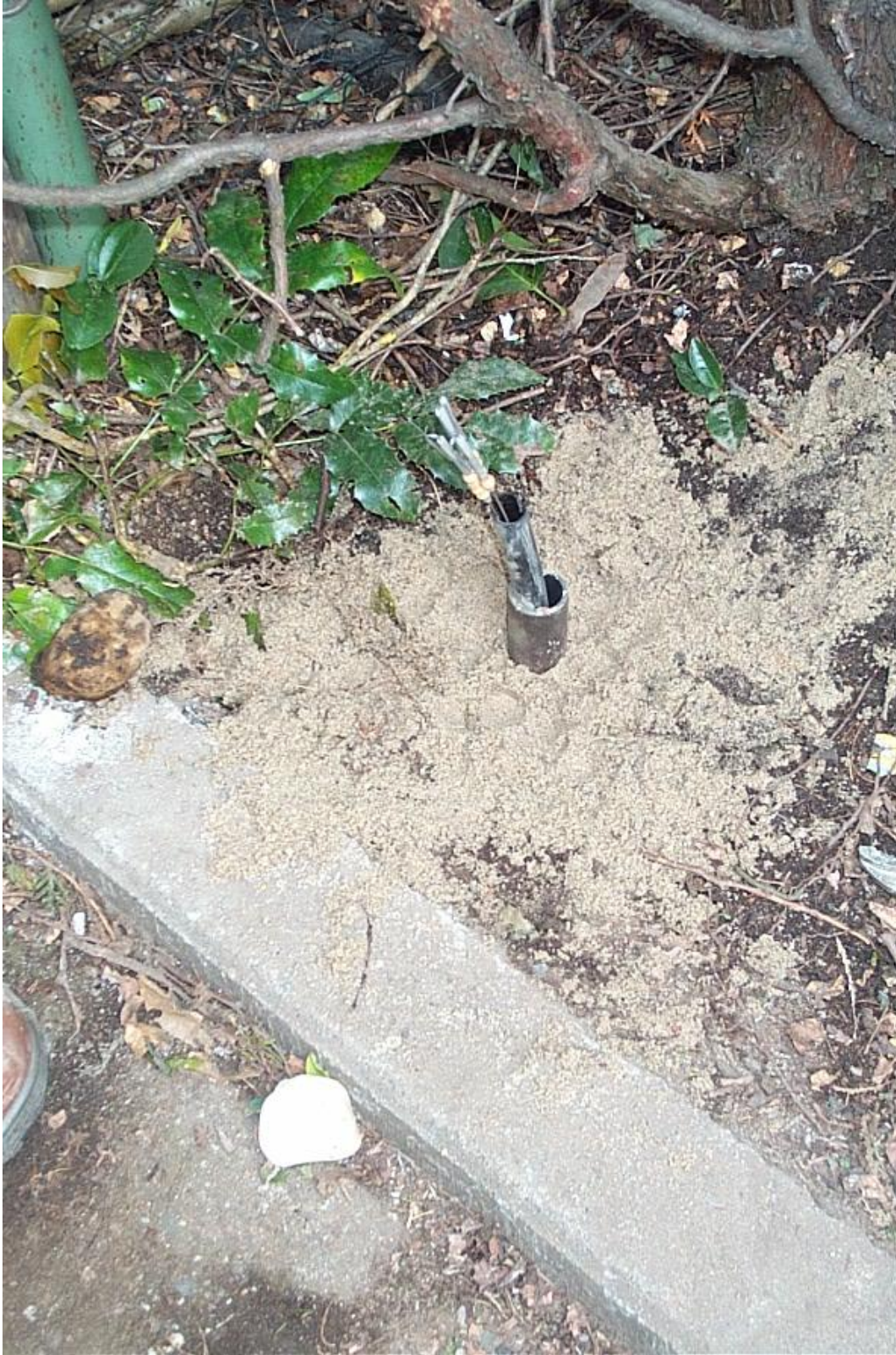
Inner protective surface casing has been installed.
