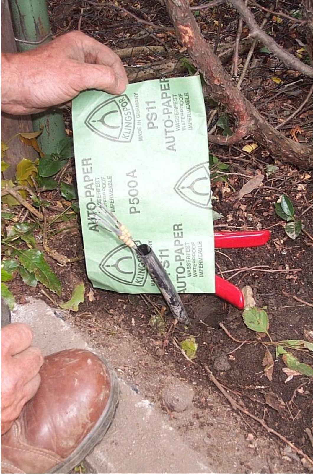
Small-diameter installation casing has been drawn. Protective tube is shown (see Figure 6).
