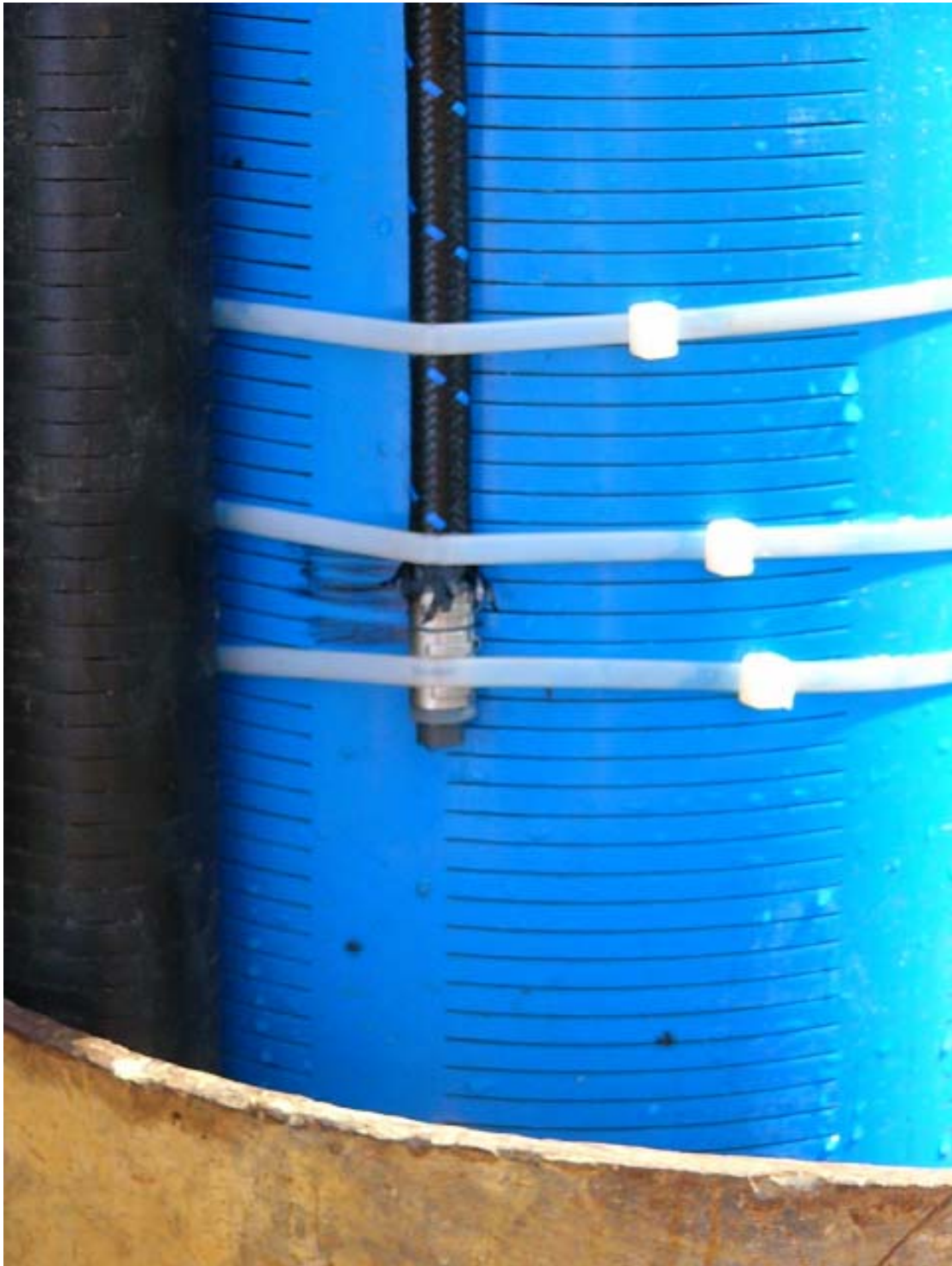
Bottom of GASSYS tube (black/blue) attached to screen of a remediation well (blue) with nearby screen of 2" piezometer (black).
