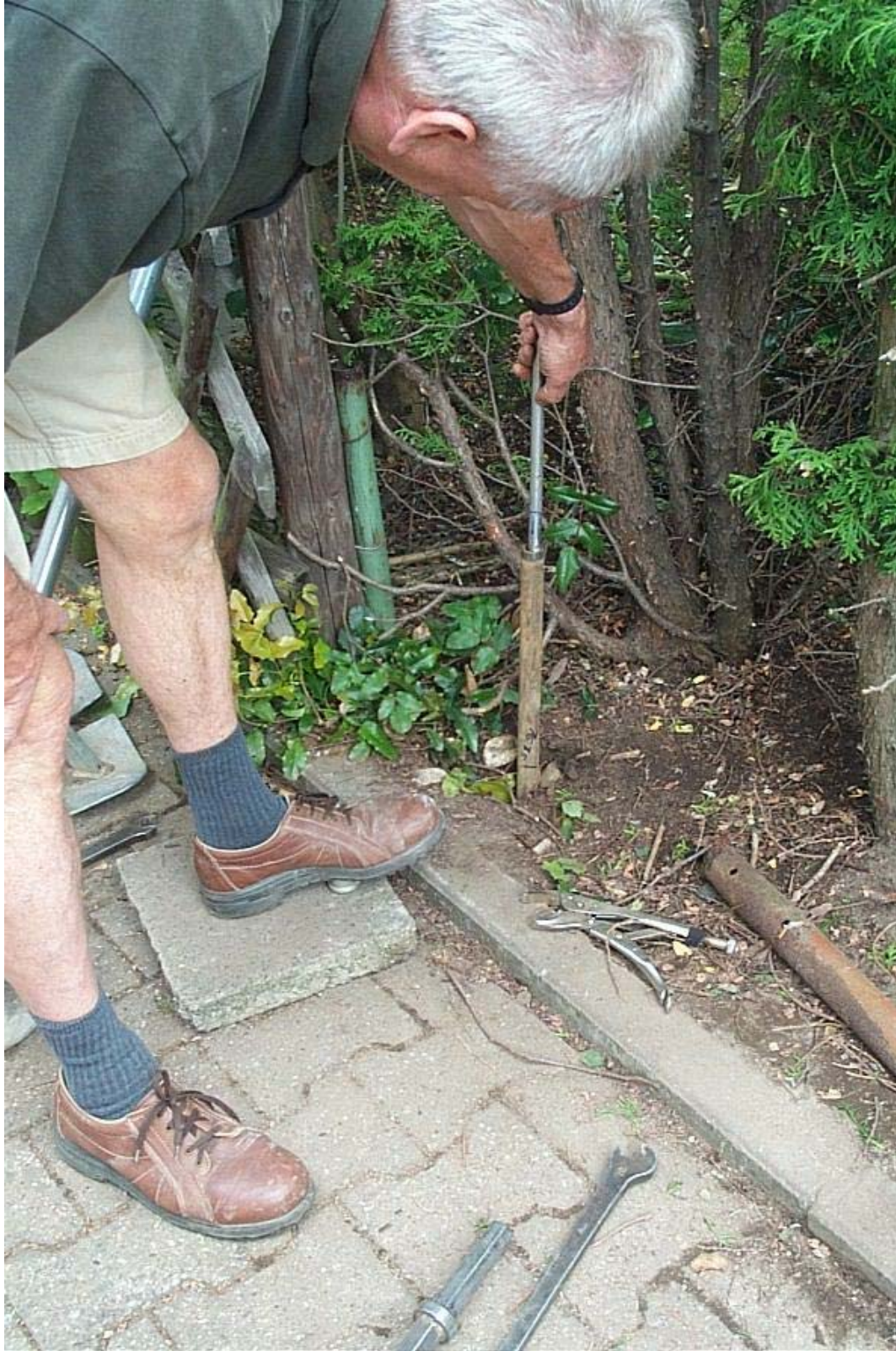
Removal of lost tip of the installation casing.
