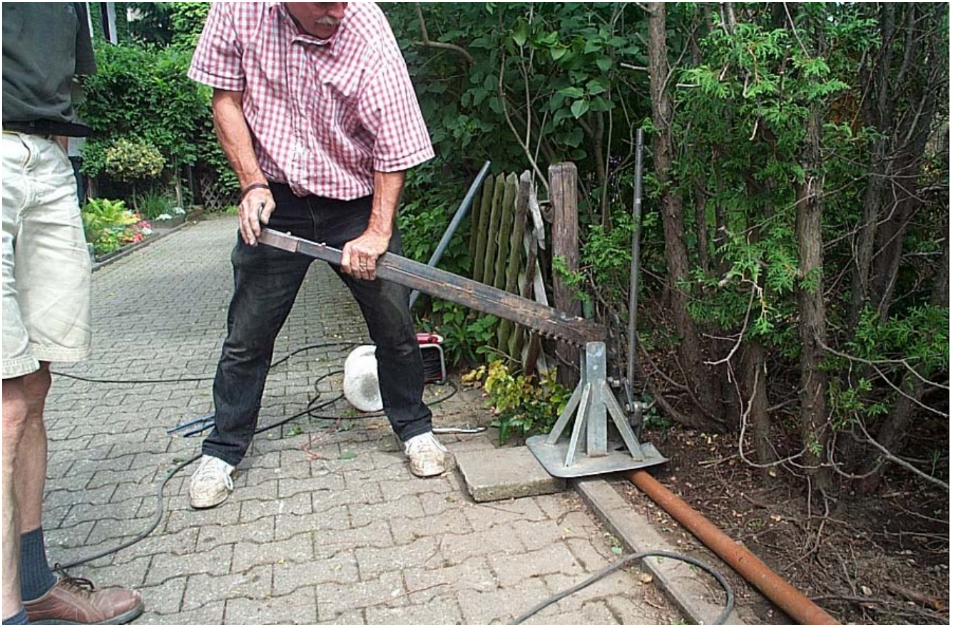
Pulling of the installation casing. Installed GASSYS hose remains in place.
