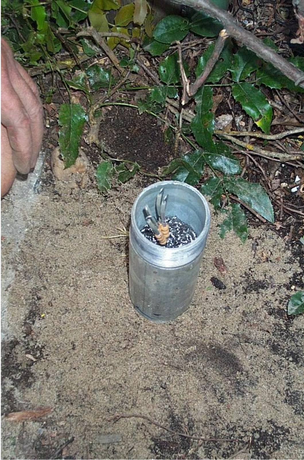
Outer protective surface casing has been installed.
