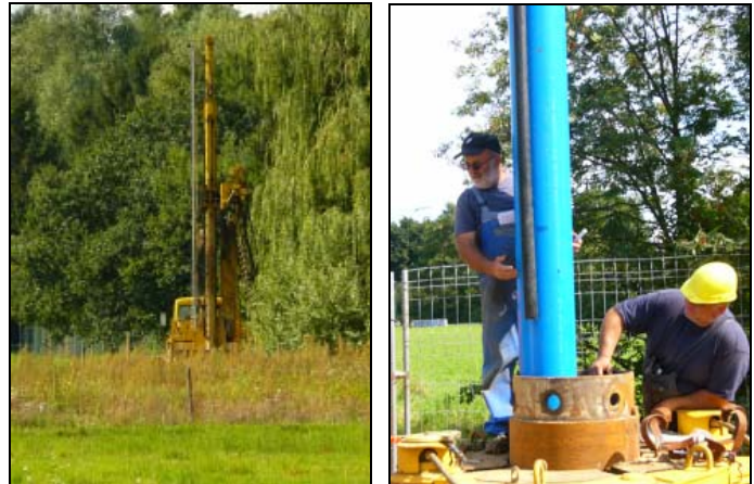
Installation of 2"-piezometer and 24"-remediation well
