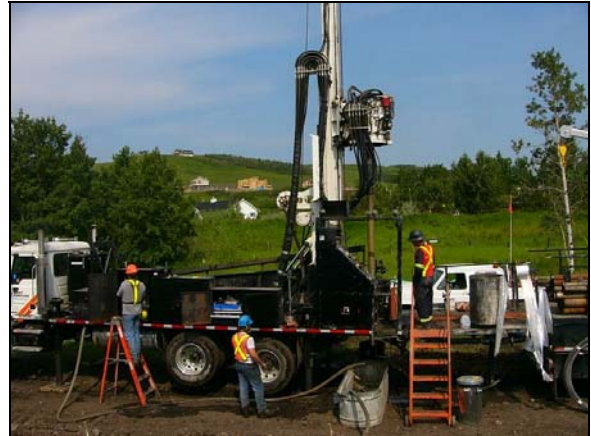
Installation of 2"-piezometers using sonic drill
