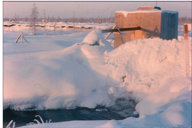
Dewatering, Pine Point Mines
