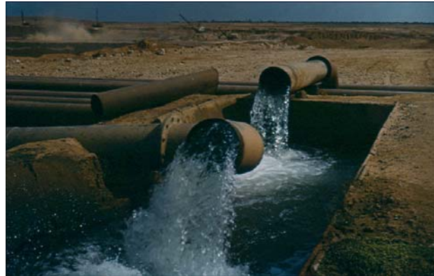
Ground water discharged by submersible pumps.
