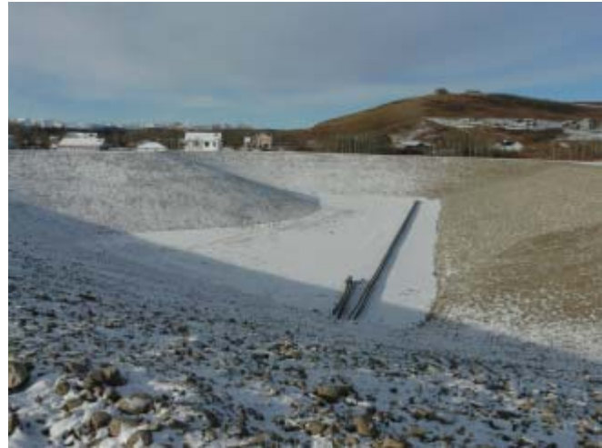
One of two water reservoirs for water supply of the Town of Turner Valley
