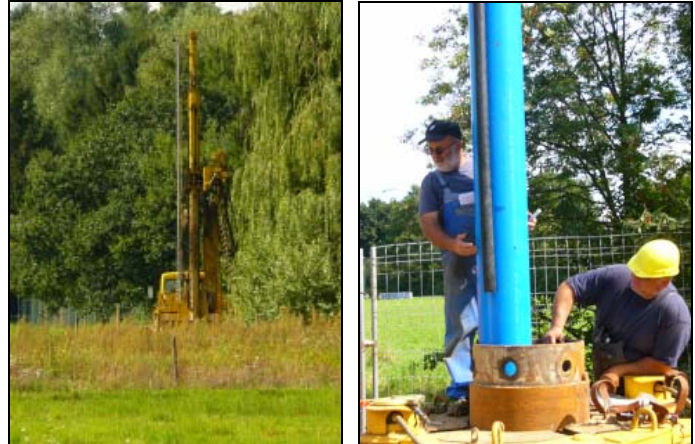
Installation of 2"-piezometer and 24"-remediation well
